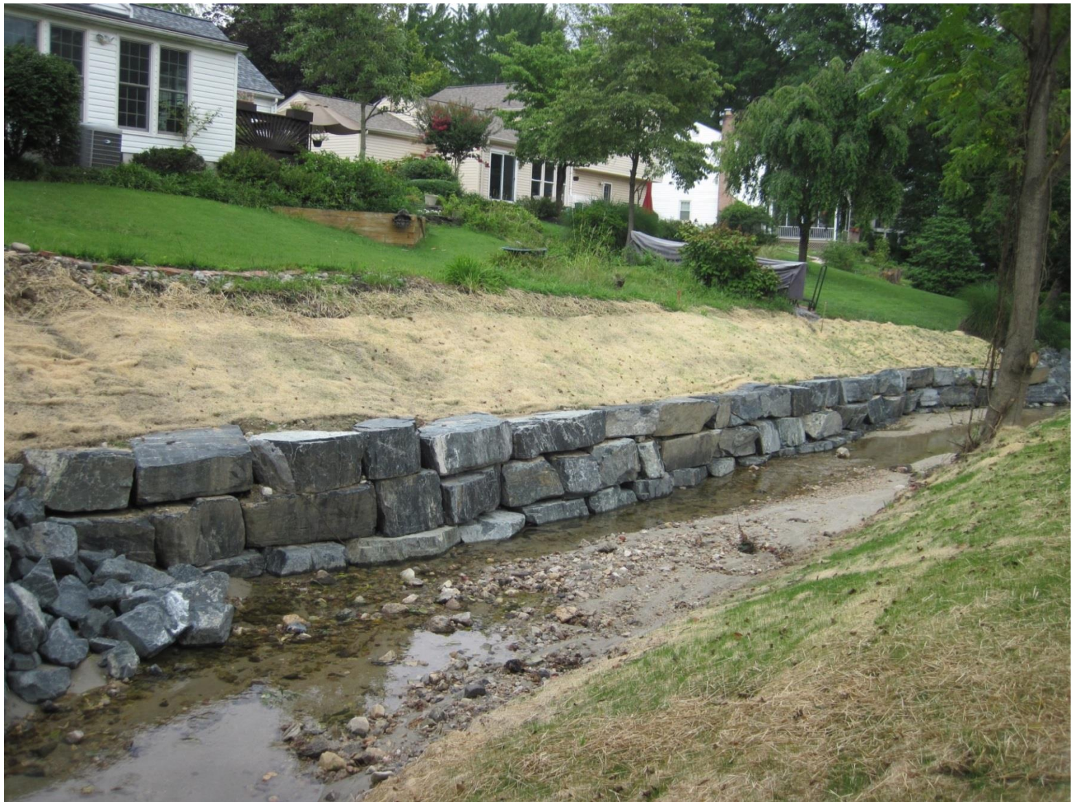
Imbricated wall behind Whetstone Rd.. Eroded bank was 34 ft. from the House. Built in 2018 Cost $35,000
