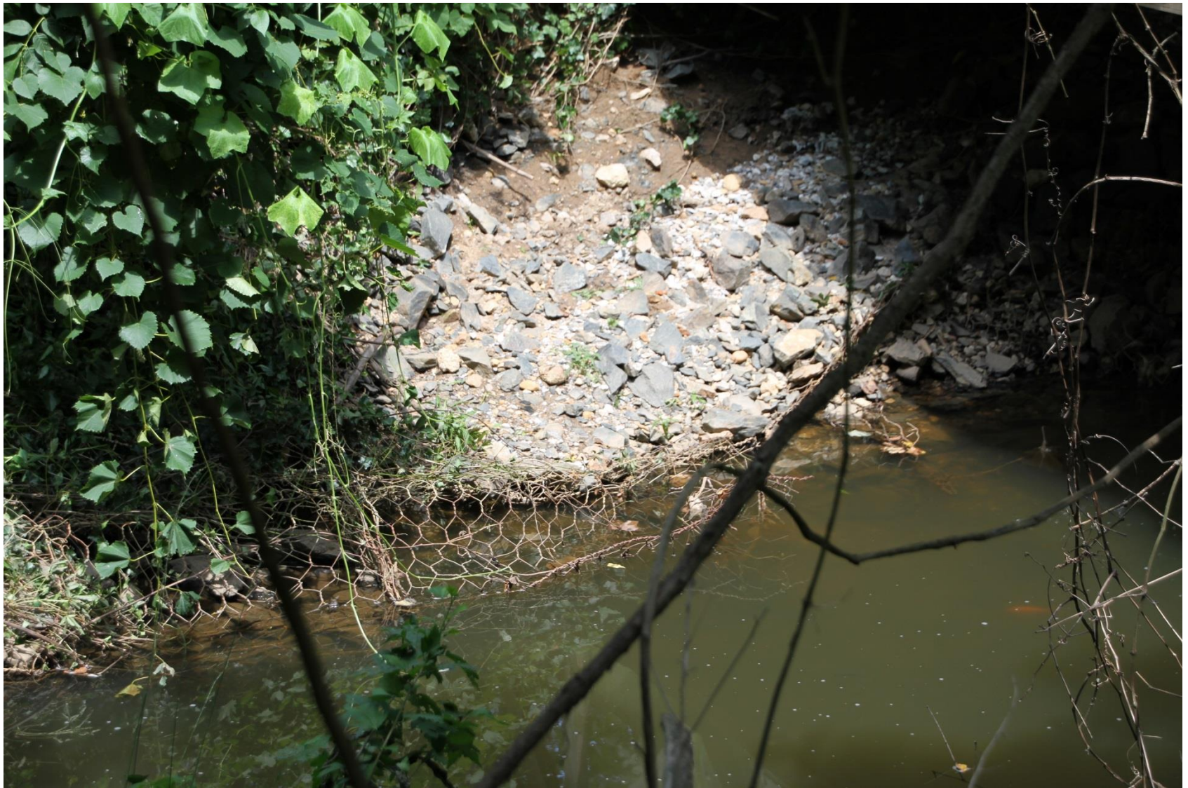
The remnants of the gabion rock baskets that were protecting the footers of the pathway bridge below the Wilde Lake dam.
