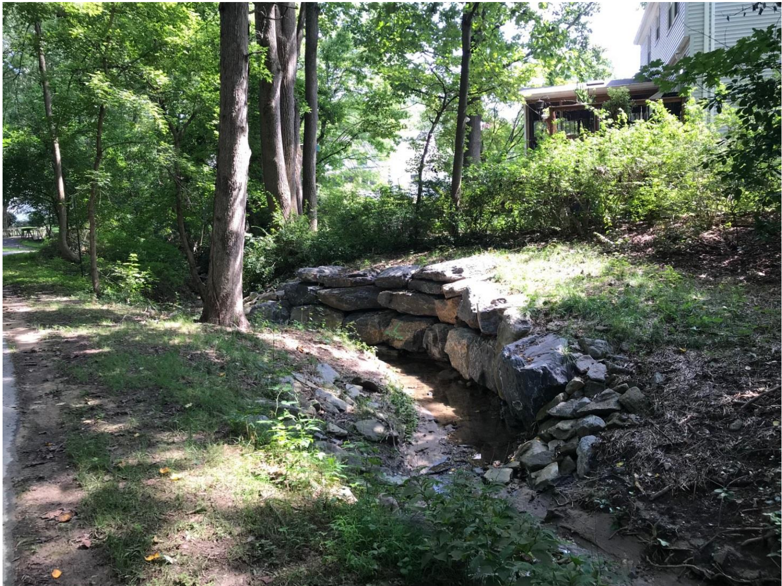
Imbricated wall behind New Leaf Ct. Eroded bank was 25 ft. from the House. Built in 2017, Cost $40,000.
