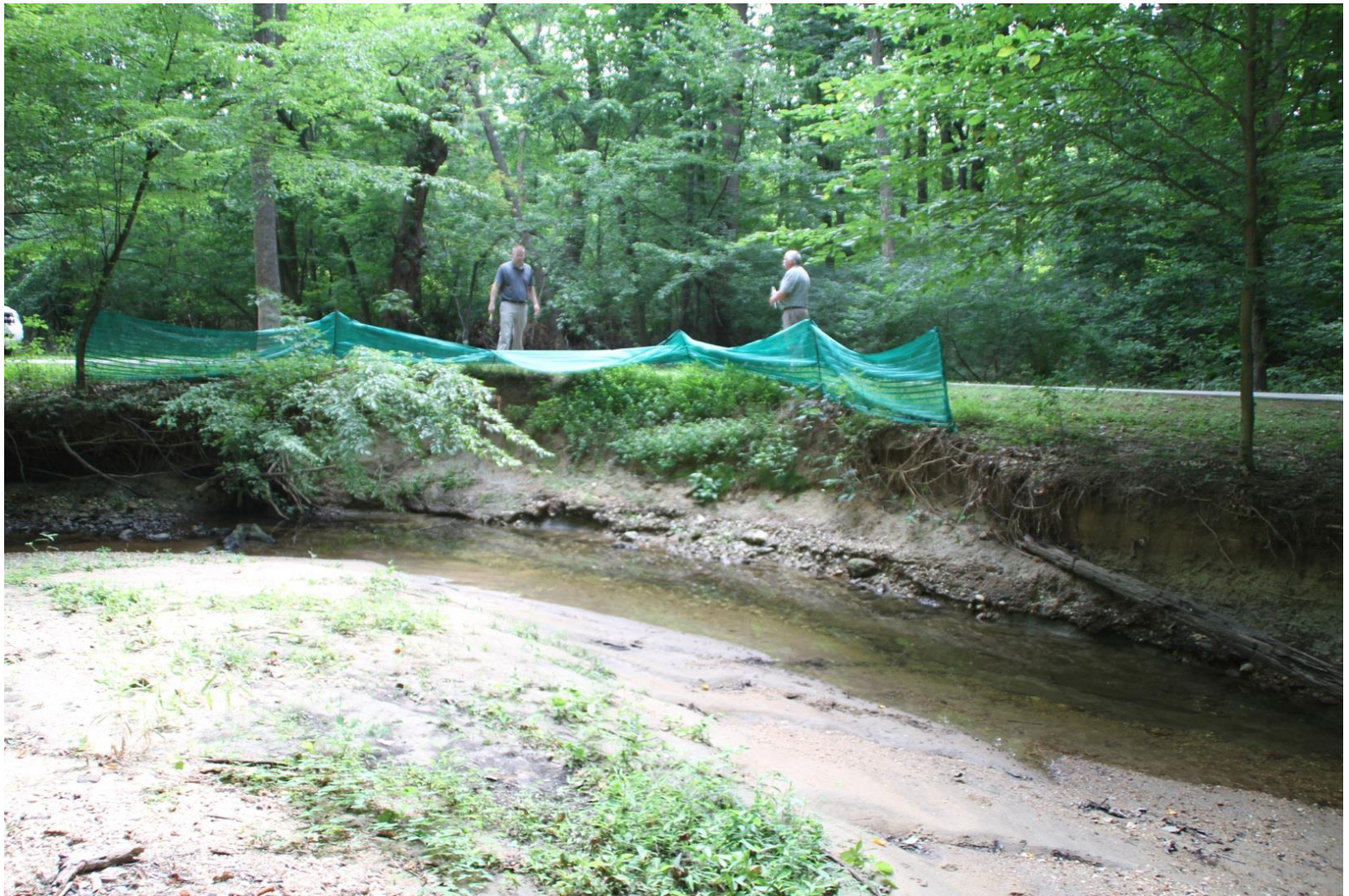
Stream bank eroding into the pathway at Footed Ridge, in Long Reach. Cost 2020 budget estimate $75,000.
