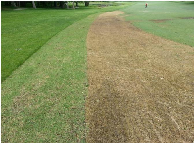
The turnhouse sewer line installation is nearing completion. The line runs the entire left side of hole # 10. The trench has been back-filled and strawed as temporary stabilization. My staff will take over soon to perform the final grading, sodding and hydro seeding. A machine, known as a rock hound will be needed to reestablish the area back to previous form. The contractor will provide a credit back to the Maintenance department for completing the work.
